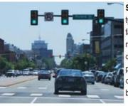
Signalized Intersection: The most common type of signalized intersection with high driver familiarity. Signal could be simple two-phase or more complex 8-phase to serve vehicular demand. Left turns can be permitted or protected (or combination of both). At a conventional 4-leg intersection there are 32 baseline conflict points.
